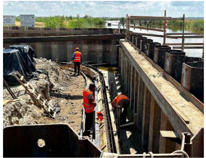
A bridge restoration in the Odesa region
