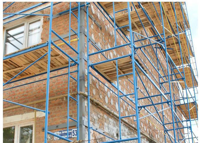
An apartment house restoration in Trostianets, the Sumy region
