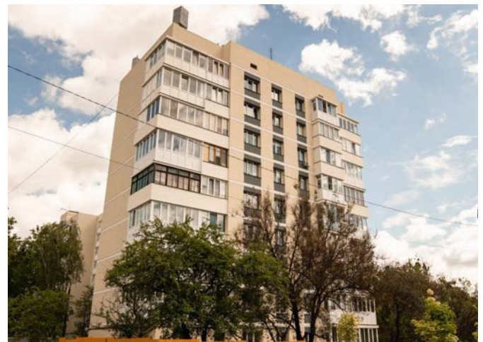
An apartment house restoration in Bucha, the Kyiv region
