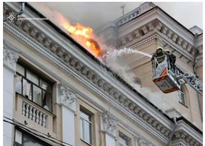
Destroyed apartment building after Russian missile attack in Dnipro
