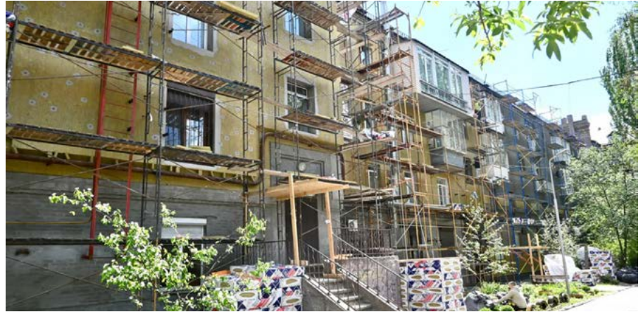
An apartment house restoration in Zaporizhzhia
